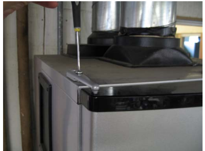
002 Unscrew the 2 fittings at the top plate. 002 Beschlag oben abschrauben 2 Stck.
